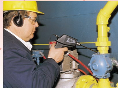
Ultraprobe 100 testing pump valve leaks
